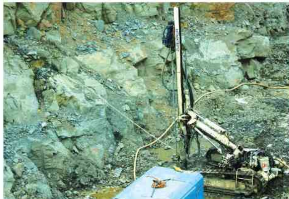
Drilling for Excavation Sangkup Irrigatin Project
