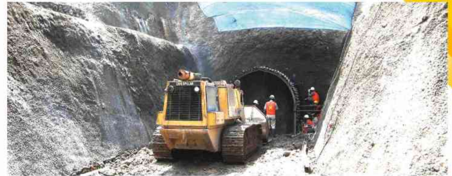
Ponre-Ponre Dam Drilling for Excavation, Bone-South Sulawesi
