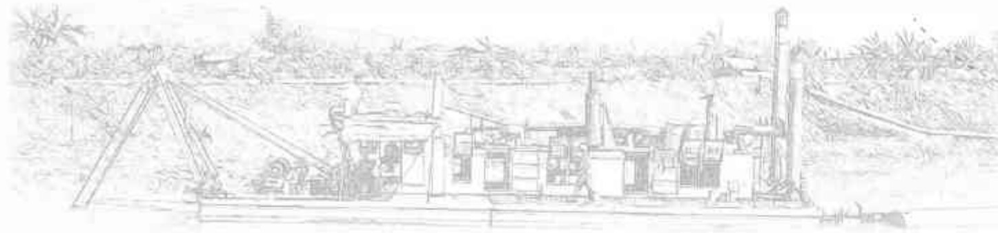
Wlingi Reservoir Work, Blitar-East Java
