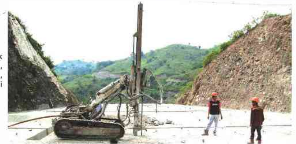
Drilling Works for Rock Anchor Bar at Spillway, Ponre-ponre Dam, Bone-South Sulawesi
