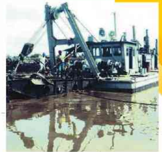
Sutami Dam Reservoir, Malang-East Java
