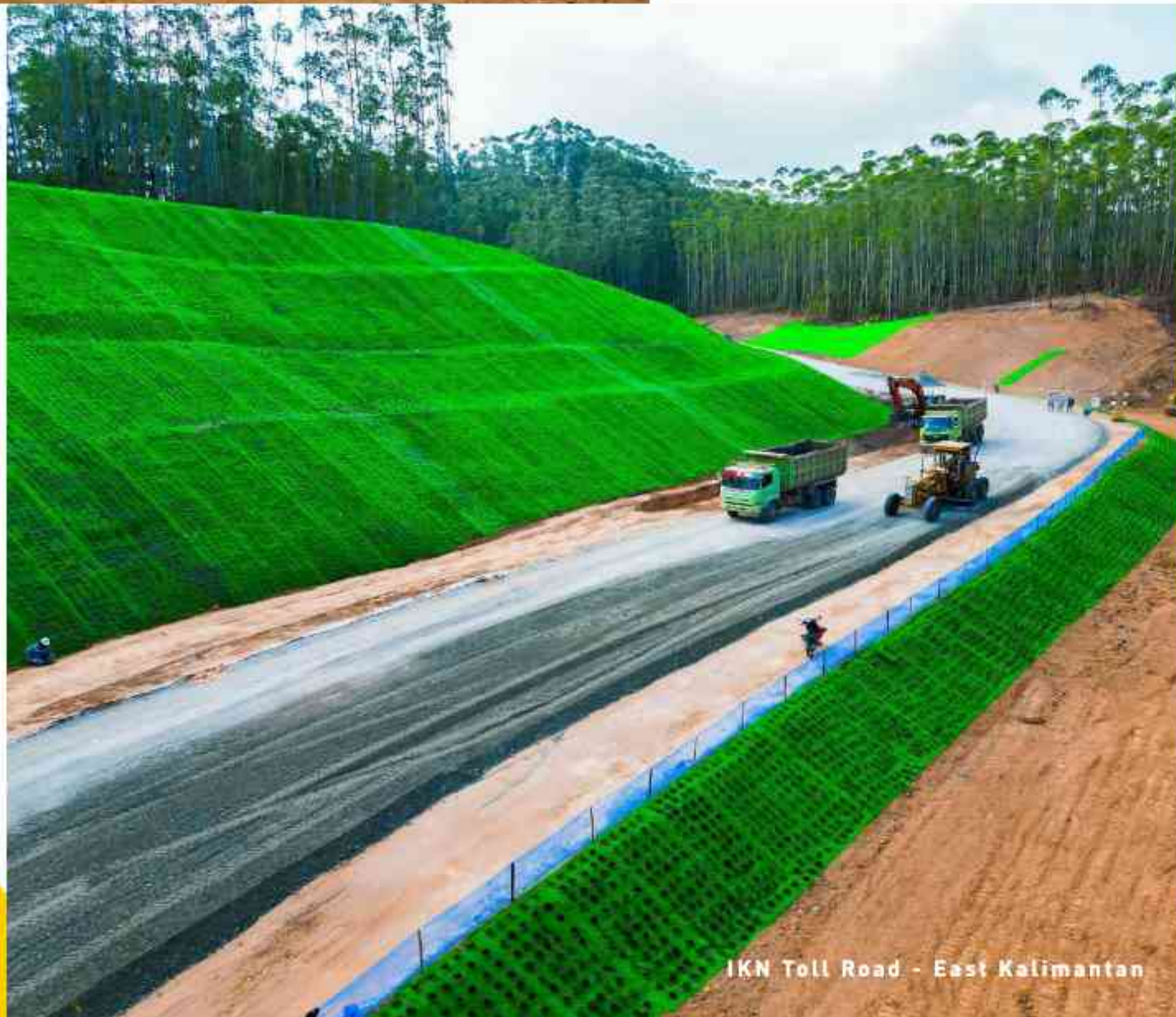
IKN Toll Road - East Kalimantan
