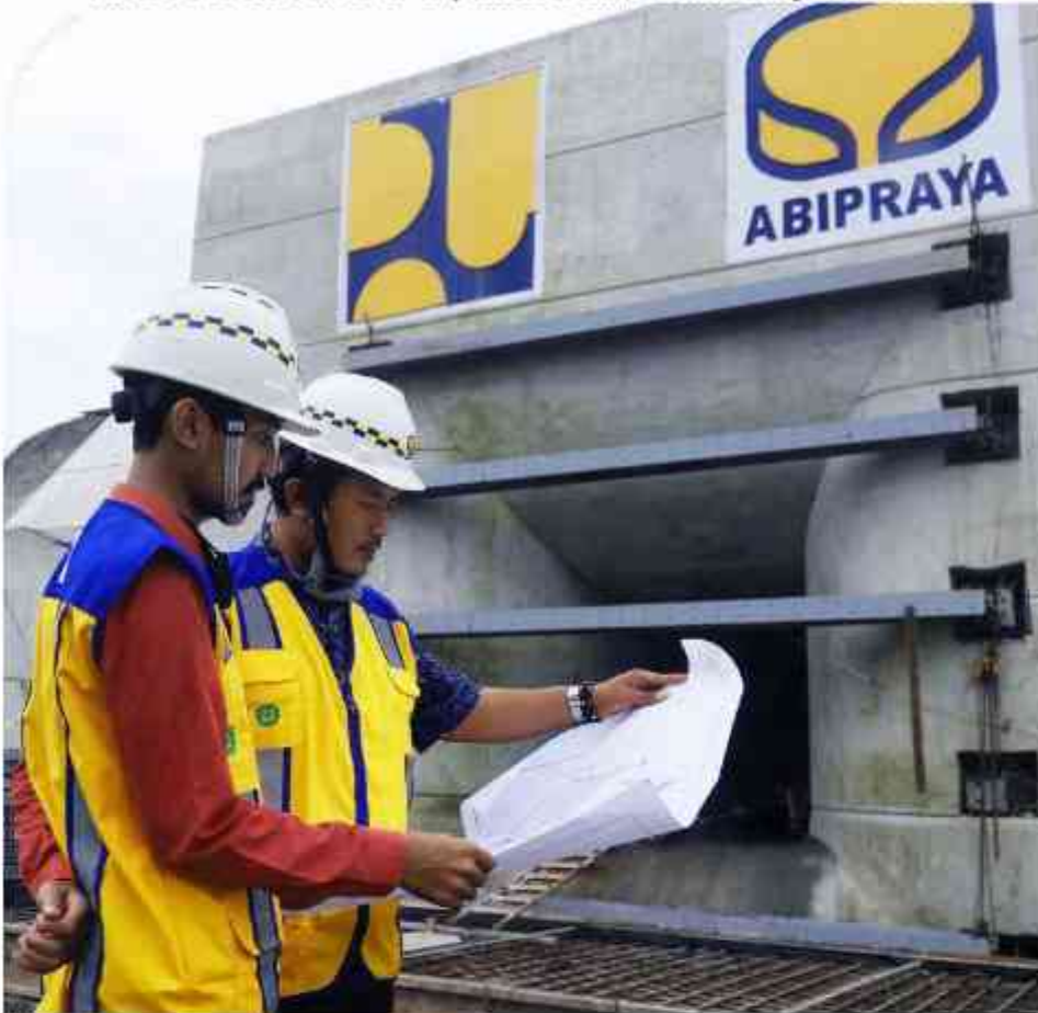
Inlet & Shaft Intake Cipanas Dam, Sumedang-West Java
