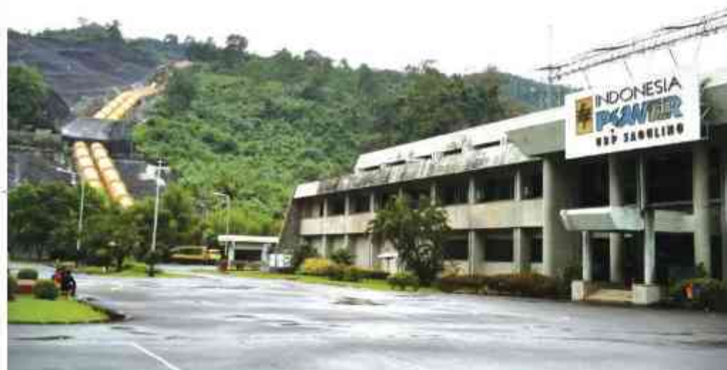
Saguling Hydro Electric Power Plant, Bandung-West Java
