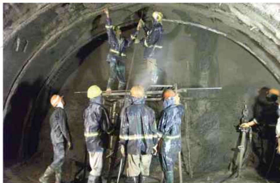
Drilling for Rock Bolt, Ponre-Ponre Dam, Bone-South sulawesi
