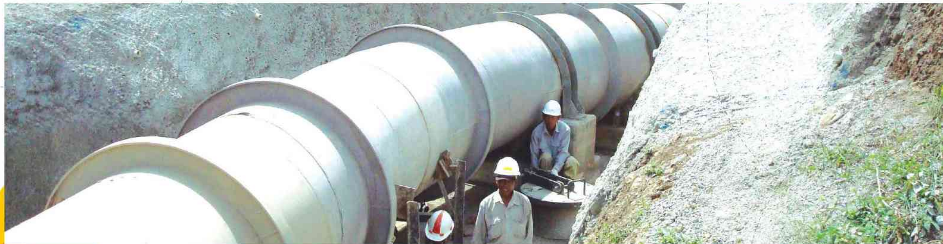
Syphon Construction of Ponre-Ponre Dam, Bone-South Sulawesi
