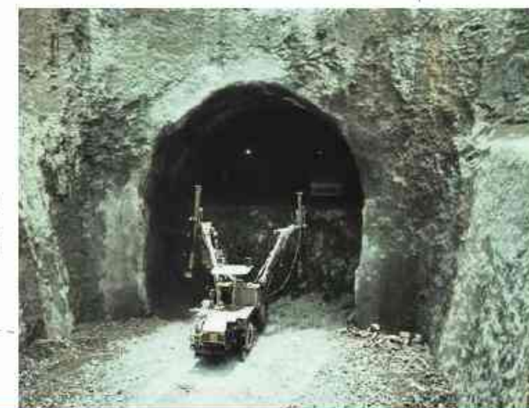
Drilling for Excavation Diversion Tunnel of the Kotapanjang Dam, Kampar-Riau
