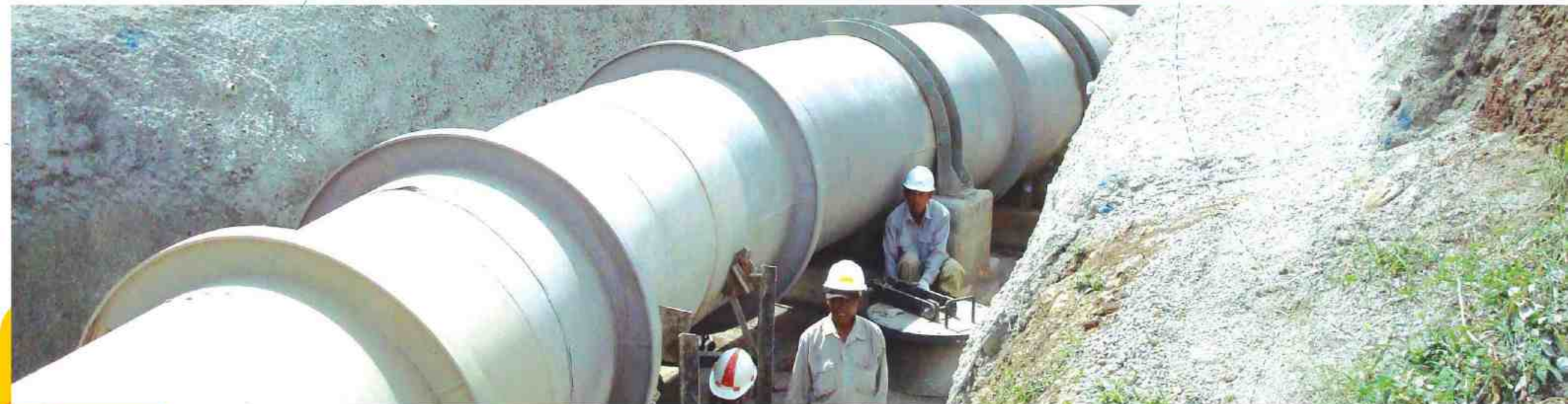
Syphon Construction of Ponre-Ponre Dam, Bone-South Sulawesi
