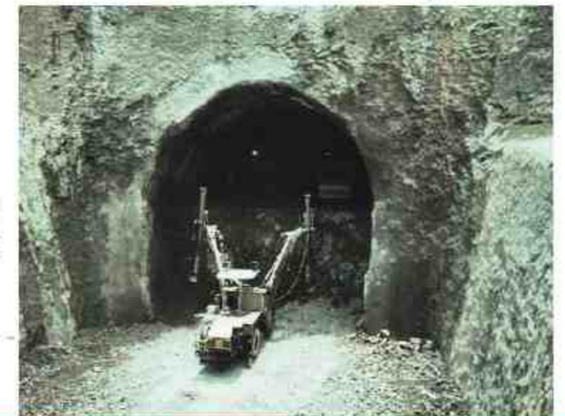
Drilling for Excavation Diversion Tunnel of the Kotapanjang Dam, Kampar-Riau
