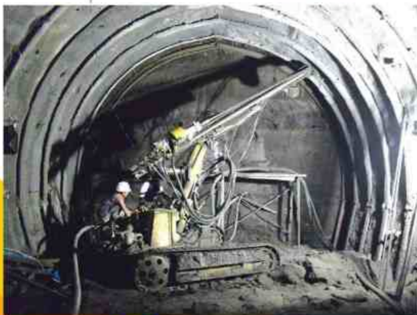
Drilling for Rock Bolt, Ponre-Ponre Dam, Bone-South Sulawesi
