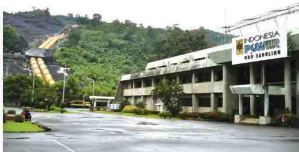
Saguling Hydro Electric Power Plant, Bandung-West Java
