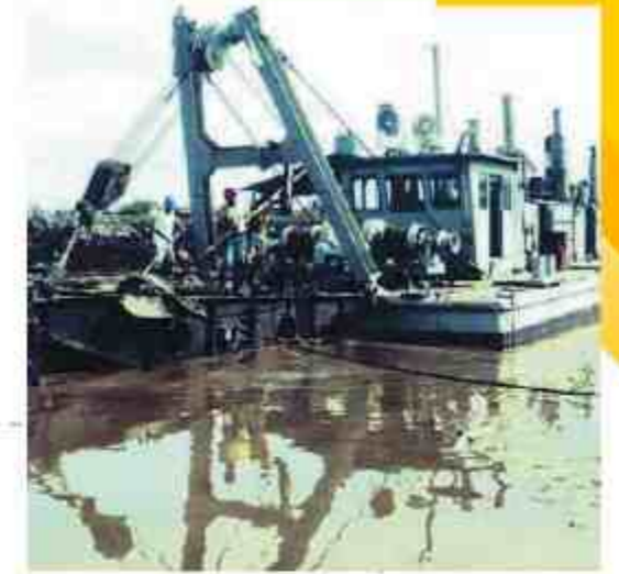
Sutami Dam Reservoir, Malang-East Java
