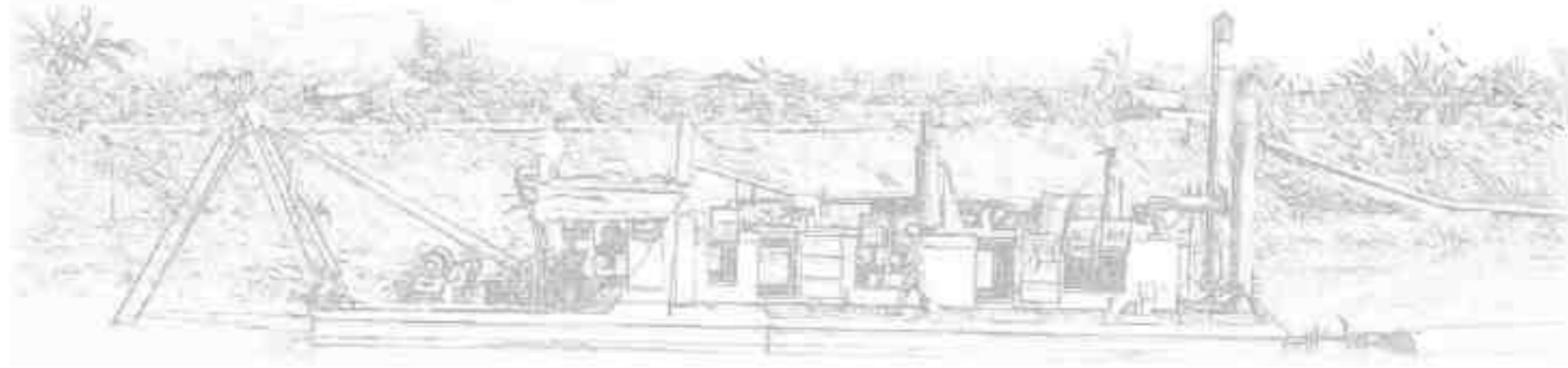
Wlingi Reservoir Work, Blitar-East Java
