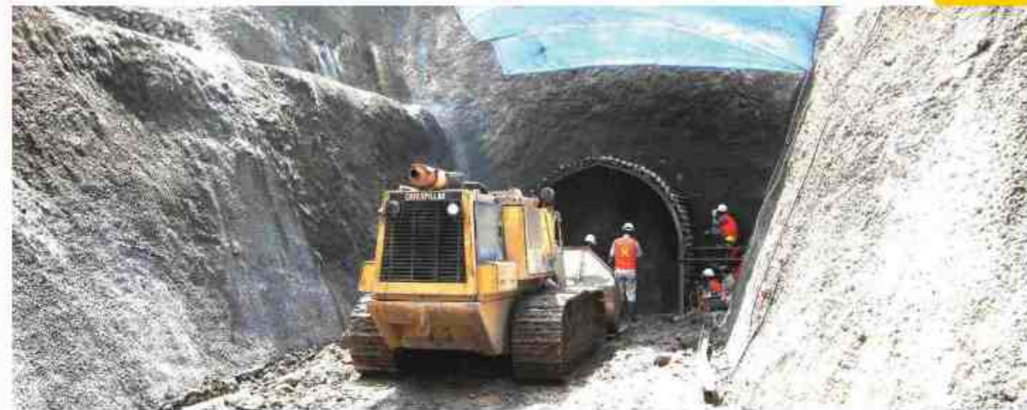
Ponre-Ponre Dam Drilling for Excavation, Bone-South Sulawesi
