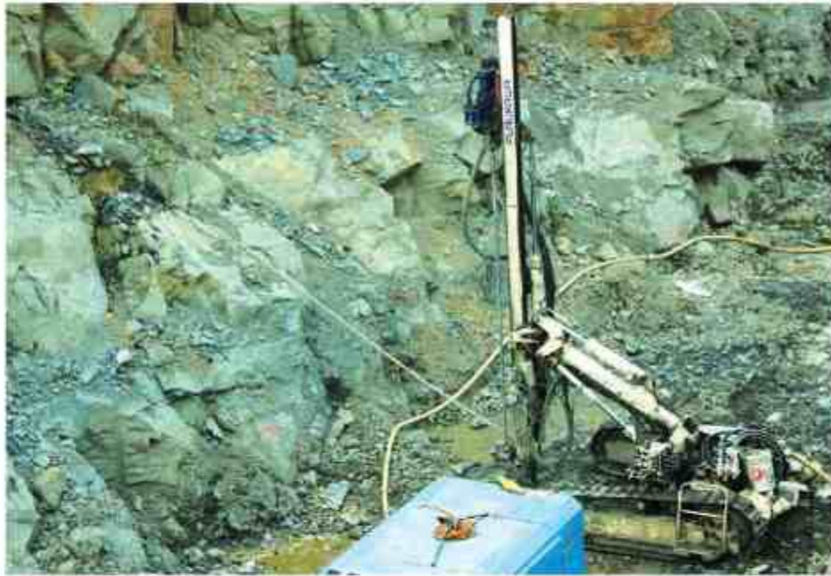
Drilling for Excavation Sangkup Irrigatin Project
