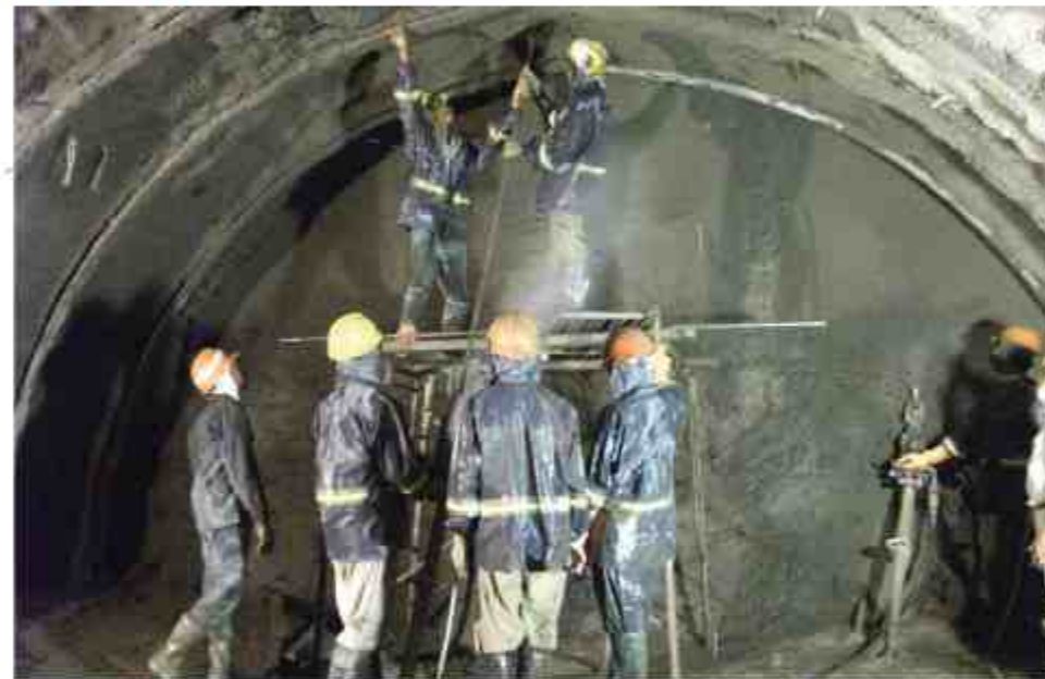
Drilling for Rock Bolt, Ponre-Ponre Dam, Bone-South Sulawesi
