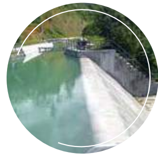
PRAFI MICRO HYDRO POWER PLANT
