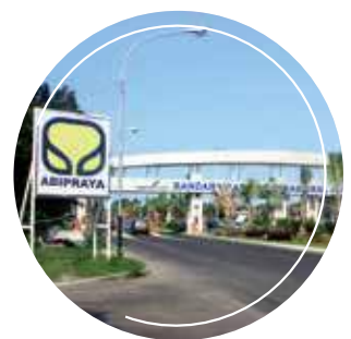
JUANDA TERMINAL 2 AIRPORT
