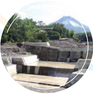
MERAPI MOUNTAIN SABO DAM CONSTRUCTION
