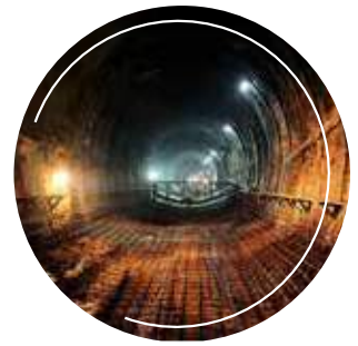
JATIBARANG DIVERSION TUNNEL
