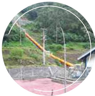
SANTONG MICRO HYDRO POWER PLANT
