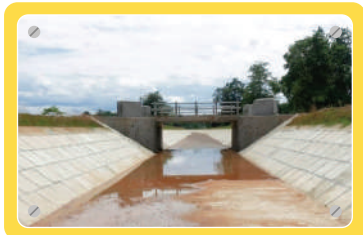
Proyek Jaringan Irigasi Baliase, Abipraya menerima Penghargaan Zero Accident dari Pemprove Sulawesi Selatan Baliase Irrigation Network Project, Abipraya received Zero Accident Award from South Sulawesi Provincial Government
